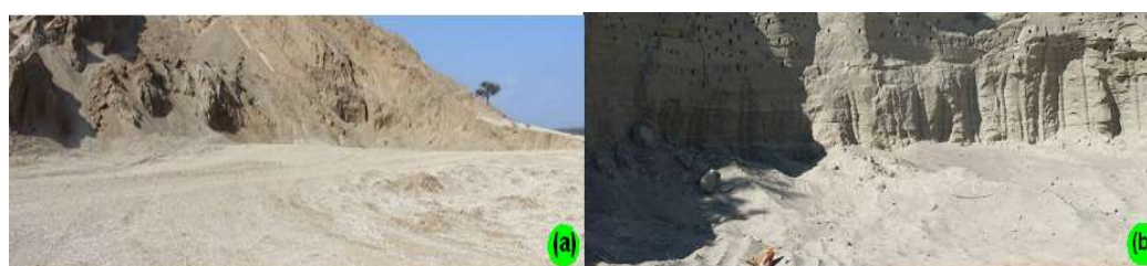
Figure 4. Illustration of the section of the magnesite (a) and copper (b) tailings that is currently being mined for different purposes at Nyala and Musina mines, respectively.
