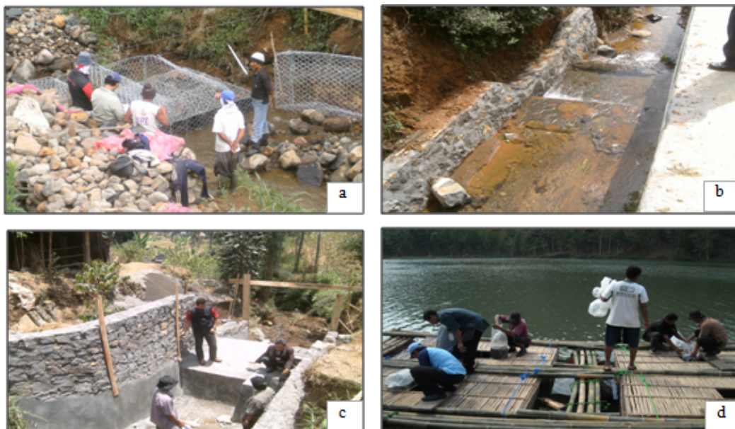
Figure 5. Small-scale dam construction from gabion (a) and stone weir (b) in Kejar Subdistrict Wonosobo Regency, rock small-scale dam in Ngadirejo Subdistrict Temanggung Regency (c) and fish cage in Kebasen Subdistrict Banyumas Regency (d)
