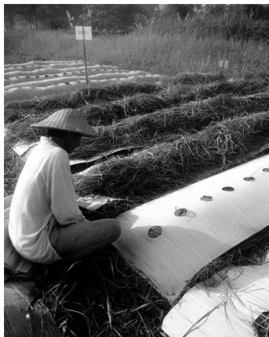
Figure 1. Biogeotextile installation
