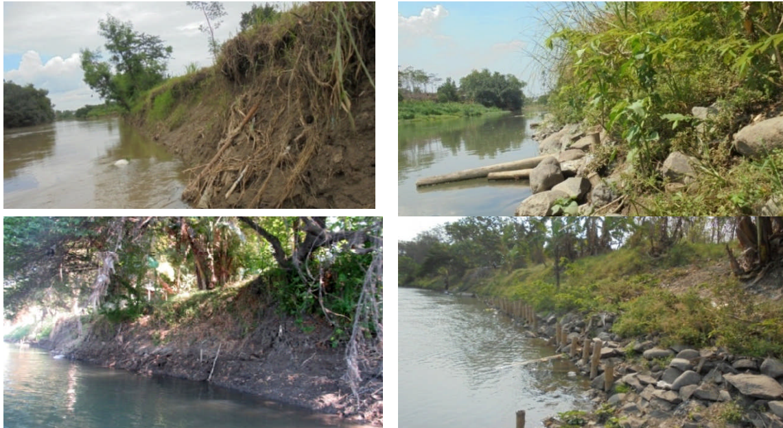
Figure 4. Riverbank condition before and after application of ECO-RIPRAP bank protection model in Wringinanom (top) and Klubuk (bottom)
