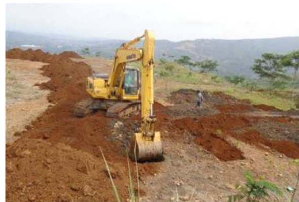
Figure 1 Application of topsoil to plant holes (Source: IPB University, 2013).
