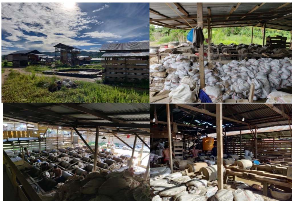
Figure 4. Processing facilities in Anggai Village, which are concentrated in one big location.
